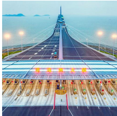
Hong Kong Zhuhai Macau Bridge
